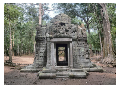
East Gate of Ta Nei Temple, Angkor after completing the full-scale restoration (Cambodia)
