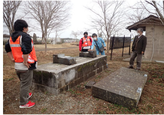
An on-the-ground survey of disaster damage
