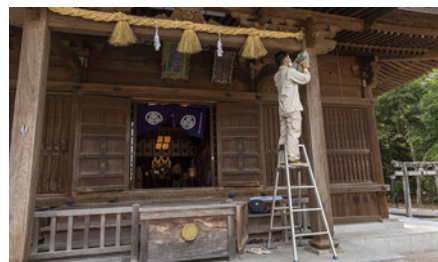
Survey of Matsue Shrine (Matsue City, Shimane Prefecture) (Nara National Research Institute for Cultural Properties)
