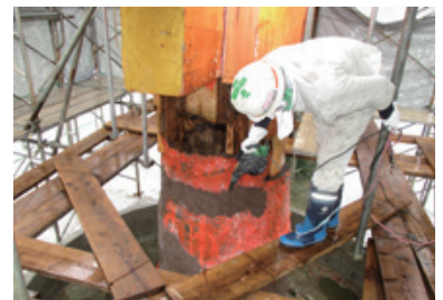
Restoration work for torii gate of Itsukushima-jinja shrine using the restoration materials, which have evaluated in this project
