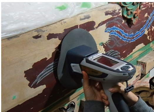
建造物の彩色調査 Investigation of paintings on a traditional building
